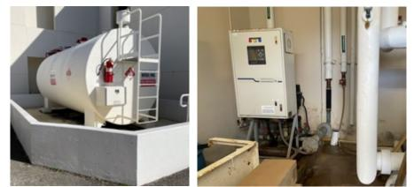
Figure 6. Examples of well-maintained generator fuel tank and pump systems.
