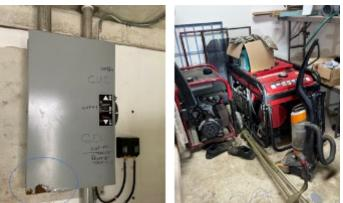
Figure 3. Examples of electrical system damage: corrosion on electrical panel (left) and nonfunctioning generators (right) see recommendation 3.
