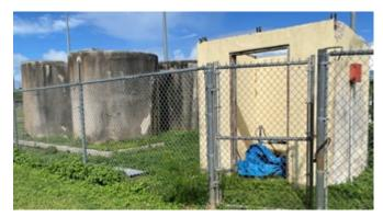
Figure 5. Examples of critical building system damage: water pump enclosure damage and water reservoir in need of maintenance.
