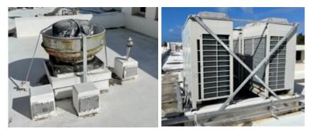
Figure 2. Examples of correctly braced HVAC rooftop units and equipment with little or no damage.
