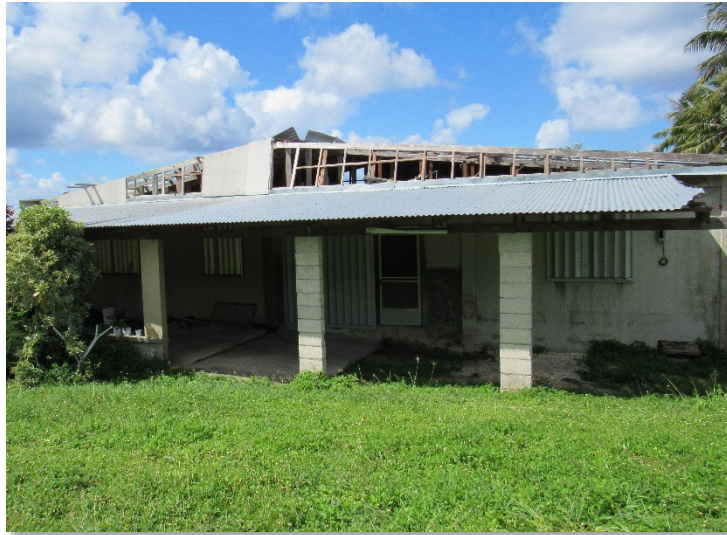
Figure 1. This photo shows a home damaged by Super Typhoon Yutu in October 2018. Strong winds blew a large portion of the roof off. The permitting and inspection process can make a home more resistant to this and other building failures. Follow this process to help protect you, your family, and your home from natural disasters.
