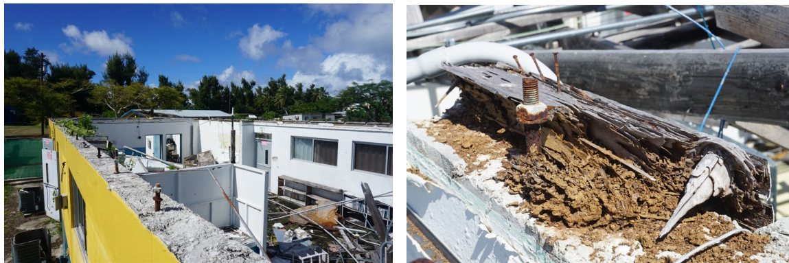
Figure 10: Left—School with compromised wooden roof trusses that caused the entire roof structure to be blown away by high winds. Right—Same school roof trusses revealing termite damage that weakened the roof-to-wall anchorage.
