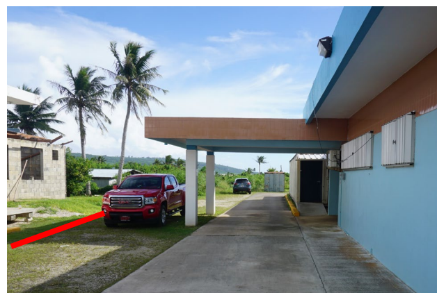
Figure 4: Left—Culvert between Tinian Fire Station and Hospital blocked by accumulated soil. Right—Hospital Emergency Entrance with canopy where surface water flowed. Design conveyance swale has filled in (red line).
