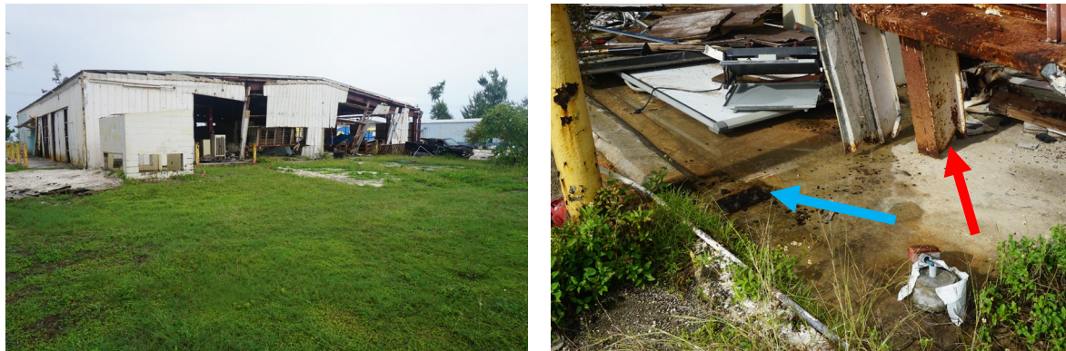
Figure 5: Left—MBS showing displaced wall. Right—Column (red arrow) at displaced wall showing corrosion of column base plate (blue arrow) and lack of housekeeping pad. Also, the building pad elevation is at grade, aggravating conditions.
