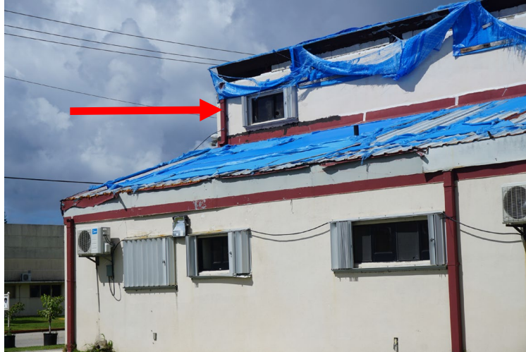
Figure 14: High window with accordion shutter that was not closed during Super Typhoon Yutu, resulting in window damage (red arrow).
