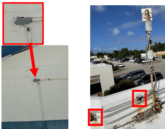
Figure 17: Left—Conduit not connected to junction; Right—Corroded junction boxes on roof of CHC.
