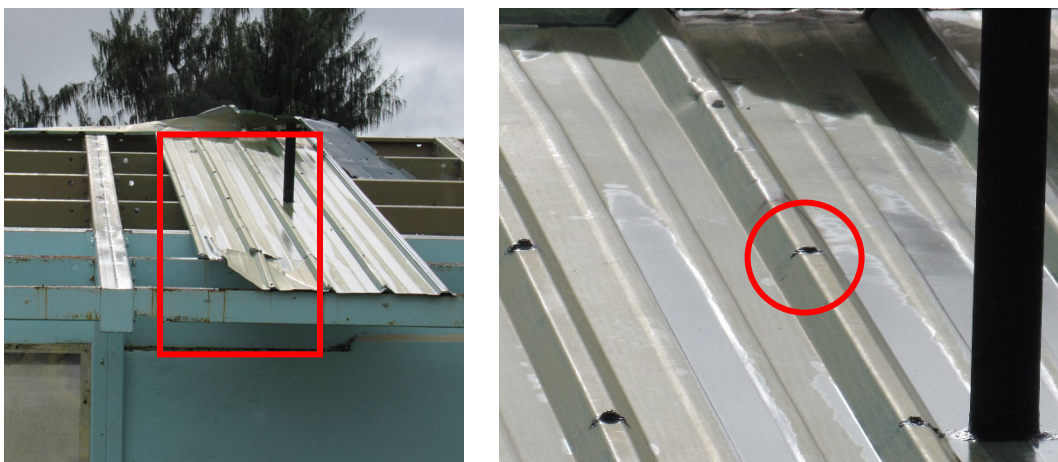
Figure 11: Left—Wind damage to metal roof with inadequate numbers and size of fasteners, Marianas High School in Saipan; Right—Closer view showing the metal roof pulled through the head of the fastener with the fastener head no longer visible.
