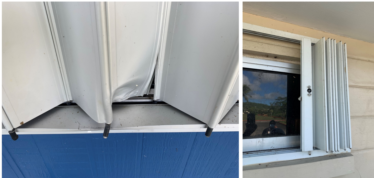
Figure 15: Left—Impact damage of non-rated, non-labeled shutter. Right—Single twist lock handle on shutters.
