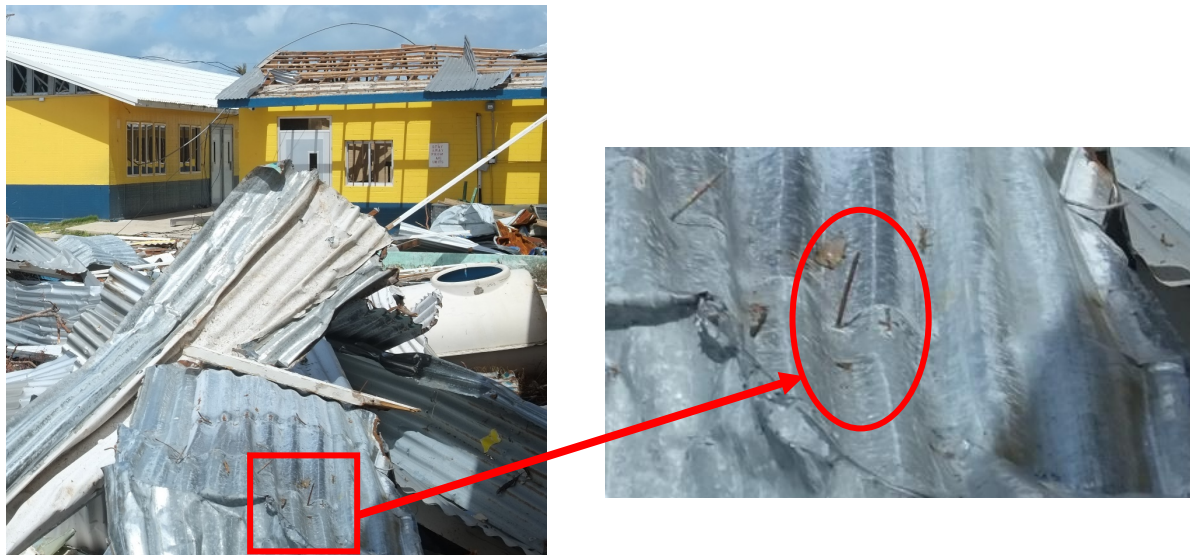
Figure 12: Left—Wind damage to Hopwood Middle School in Saipan; Right—Inadequate fasteners, such as nails, led to much of the damage. [Image credit: Forrest Lanning, FEMA]
