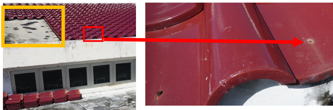
Figure 13: Left—Tile roof damaged by strong winds at the Office of Aging; Right—Corrosion of fasteners contributed to the failure.
