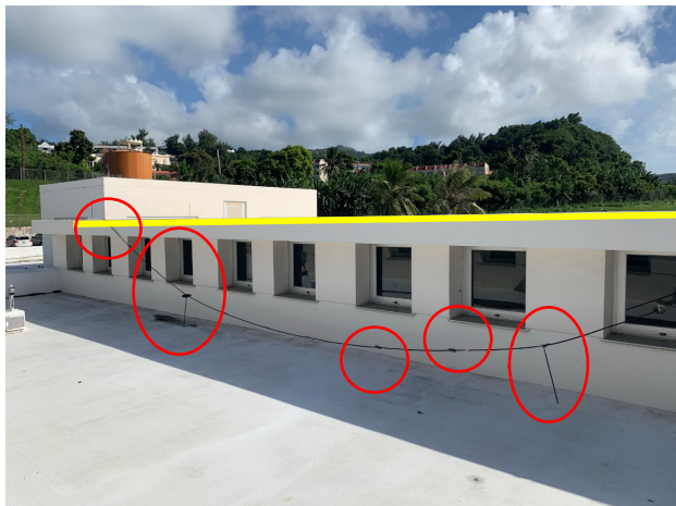
Figure 19: Failed connectors from lightning protection system. Air terminals were displaced when the system connectors failed.
