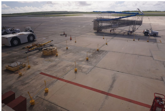
Figure 9: View of damaged passenger boarding bridge location. Original storm mooring foundations are painted yellow (left side).
