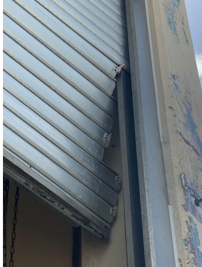
Figure 16: Damage to large, rolling door at fire station apparatus bay at Fire Station 2.
