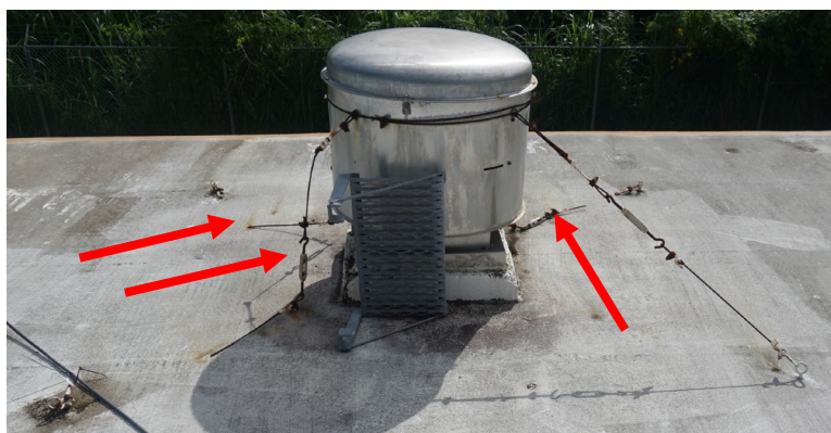
Figure 7: Rooftop fan unit where three of four cable anchors failed because of corrosion (red arrows).
