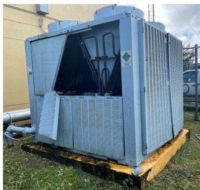
Figure 18: Emergency Operations Center, Left—Replacement mini-split units; Right—Abandoned condenser.
