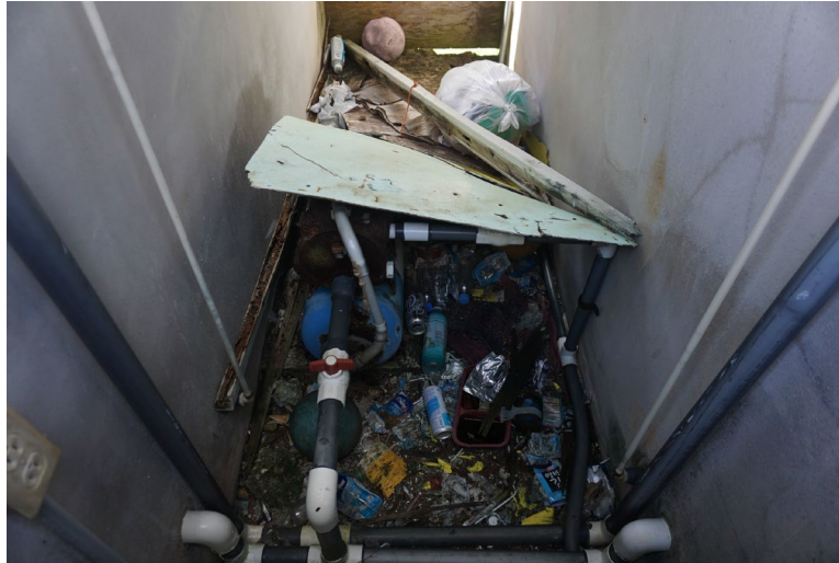
Figure 8: School water pump in building enclosure that did not provide adequate weather protection.
