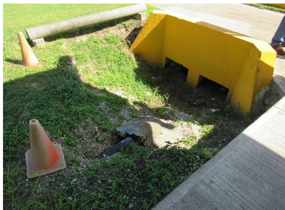
Figure 4: Left—Culvert between Tinian Fire Station and Hospital blocked by accumulated soil. Right—Hospital Emergency Entrance with canopy where surface water flowed. Design conveyance swale has filled in (red line).
