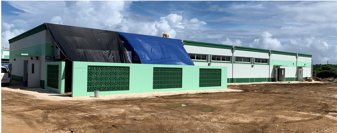
Figure 22: New cafeteria at Koblerville Elementary School identified for use as an emergency shelter, but was not designed to meet FEMA or ICC life safety protection criteria.
