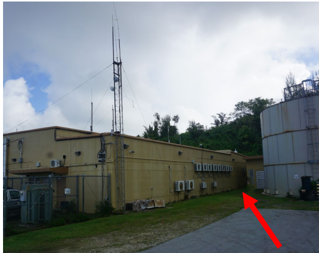
Figure 3: The architectural reveal along the side of the EOC (yellow building) is approximately 1 to 2 feet above the interior finished floor. The narrow area where drainage flows is indicated by a red arrow.
