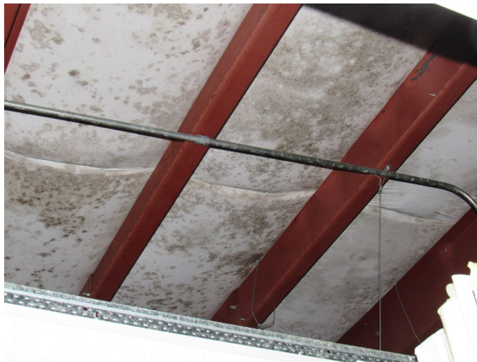
Figure 6: MBS plastic-wrapped blanket insulation showing organic growth due to inability to remove water from interior layers of insulation.
