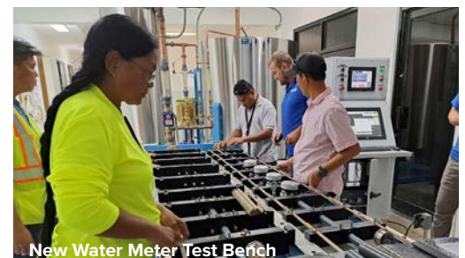
New Water Meter Test Bench
